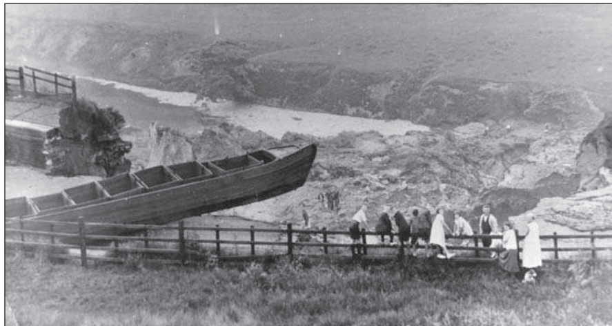
Figure 9 – The 1936 Manchester, Bolton and Bury Canal Breach
